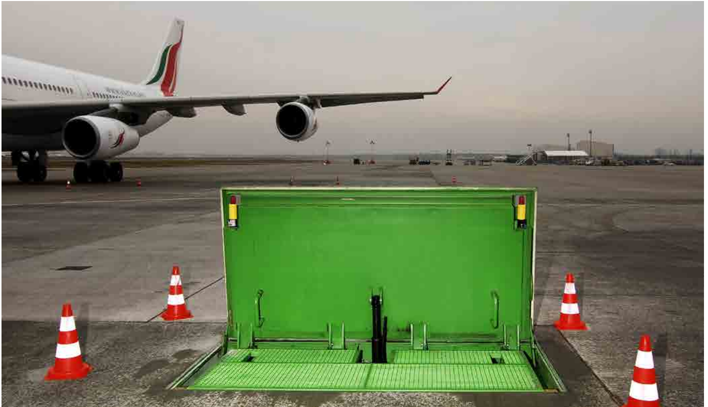
Frankfurt Am Main Airport, Frankfurt, Germany - LY Hydraulic range
