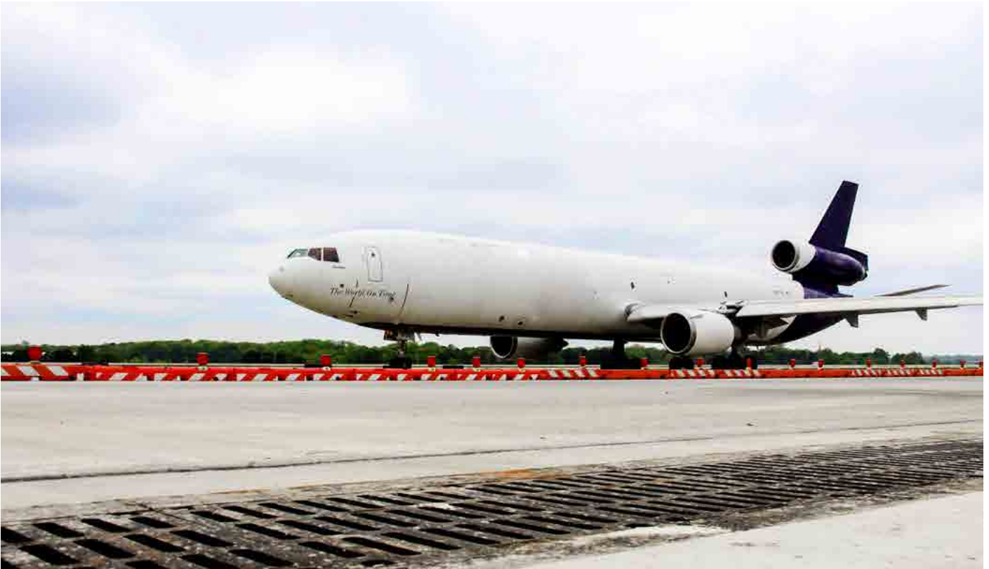
Memphis International Airport, Memphis, United States of America - Drainage range
